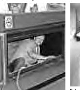
Electrician Rick Miles installs a conduit inside the terminal ticket counter
