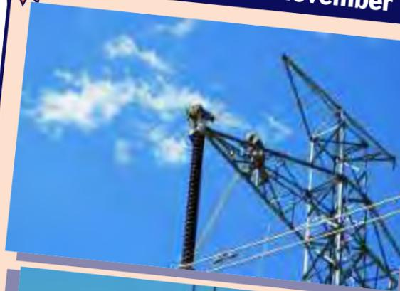
"Cooning the bells -- This tower is 135 feet tall. Cooning the bells means climbing down the insulators to the wire, then you put a spacing cart on. The spans are a quarter-mile long."
