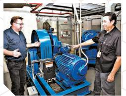
The library's elevator motors are installed in a room above the library. These units are among the newest in the City. Here (from left), Brian Teague, Elevator Mechanic (Hiring Hall) and Ramon Pasillas, Elevator Mechanic, 5 years of City service, Club Member, inspect one of the 40-horsepower motors.
