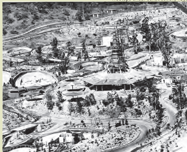
Treetops under construction, 1965.
