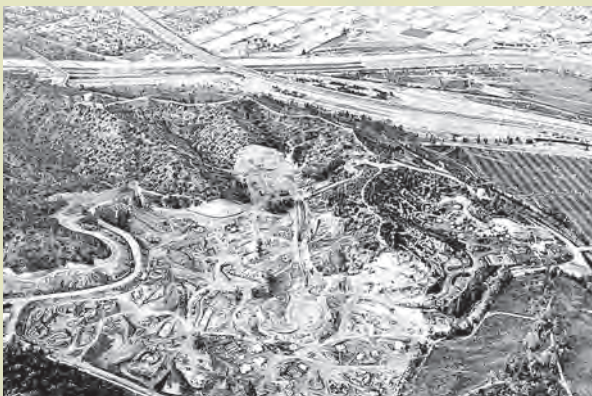
From March 1965: An aerial view of the Zoo grounds under construction. The children's zoo would be the first to open, in April 1965. The rest of the Zoo opened in November 1966.
