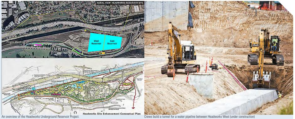
Crews build a tunnel for a water pipeline between Headworks West (under construction) and Headworks East, already in operation."
