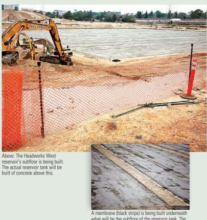
what will be the subfloor of the reservoir tank. The membrane material is basically the same as roofing material, only several times stronger
