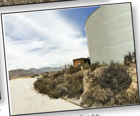
The million gallon water tank, still on duty.
