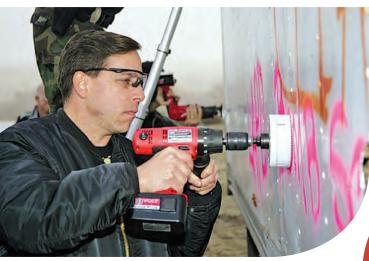
Sgt. Michael Salinaz, the Officer in Charge of the Bomb Squad, cuts through a panel truck's wall so the squad can insert a camera and examine the truck's contents.
