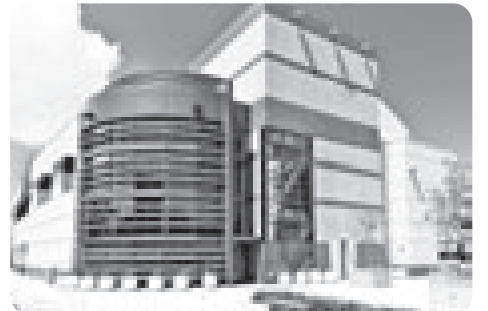
The new Port Police building is at 330 Centre St.
