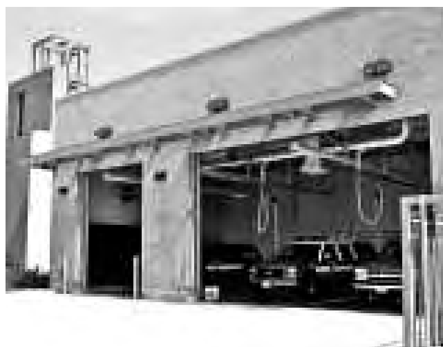
The new Fire Station 5.
