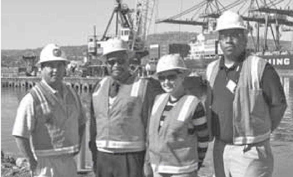
At Berth 145-157 Wharf Construction project at the Harbor were (from left) Senior Construction Inspector Michael Chung, Public Works/Contract Administration; mentee Robert J. Washington; mentee Marcia Villanueva; and Senior Construction Inspector Roosevelt Bagby II, Public Works/Contract Administration.
