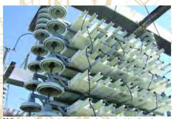
DC filters have to be cleaned every other year since the electricity collects dust onto the surface of equipment.
