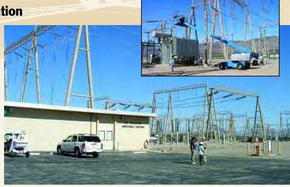
The McCullough Switching Station, south of Boulder City, gathers power from a number of sources and sends it where it's needed. Inset: Larry Jurn, Electrical Mechanic, is in the "bucket," installing a new transformer.
