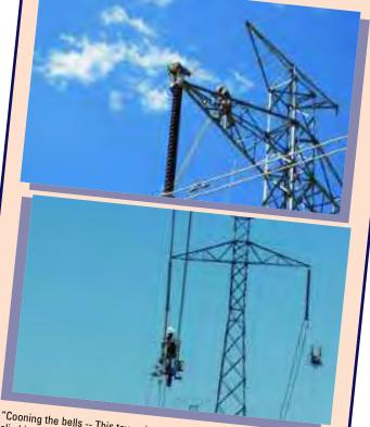
"Cooning the bells -- This tower is 135 feet tall. Cooning the bells means climbing down the insulators to the wire, then you put a spacing cart on.
