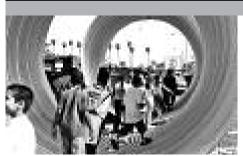
The students walk through a 14-foot-in-diameter corrugated metal pipe (CMP) that will be used to line the microtunneling shaft and protect the men working inside the shaft. Leading the students is Adrian Torres, a laborer working for subcontractor August Construction
