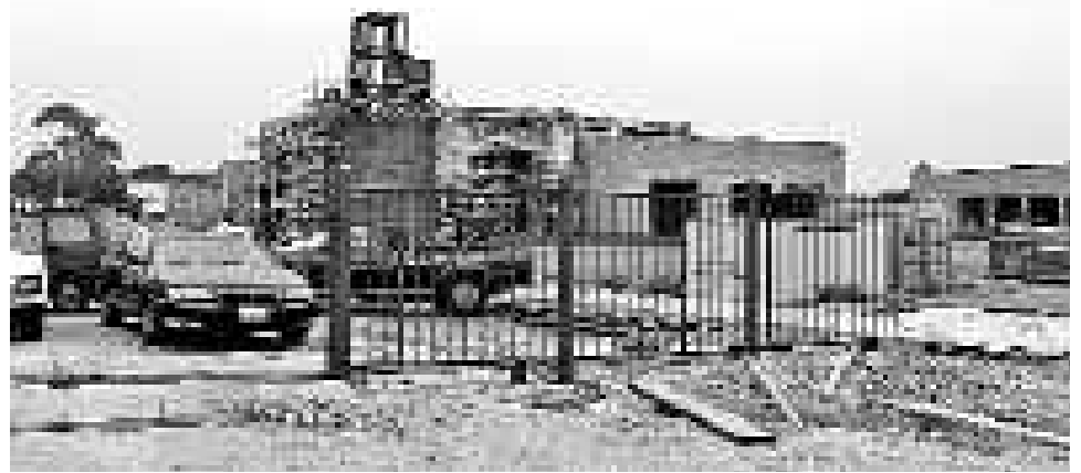
Fire Station No. 5 going up in Westchester.
