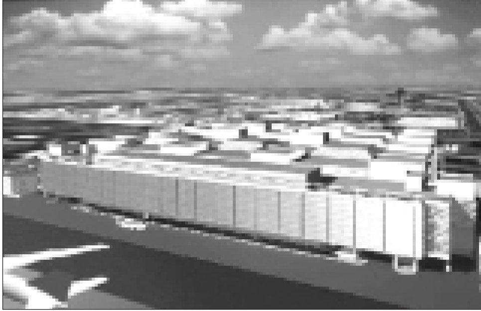
LAX's Bradley Terminal is scheduled to undergo renovation.
