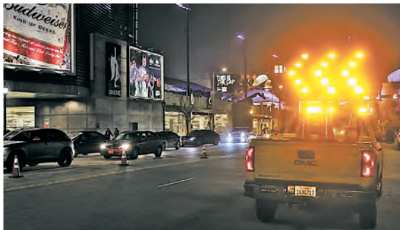
With the Kings game now over, the cones, barricades, arrow truck and specially timed signals funnel the traffic from Lot 1 (on Georgia Street) and the West Garage Gate B west toward the 110 Freeway. With the traffic devices in place, Transportation can empty the two parking lots in less than 30 minutes.
