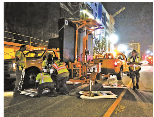
The special events crew starts its street closures around 3 a.m.
