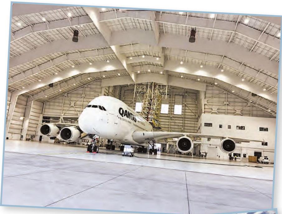
The new Qantas airplane hangar at LAX.
