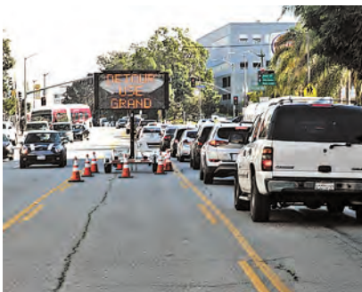
Traffic control signboards informed drivers that lanes were closed on Cesar Chavez Avenue.
