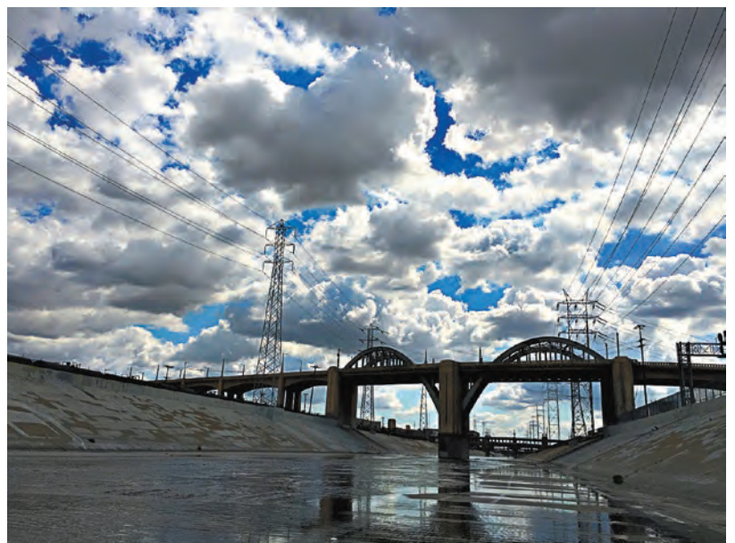
"After the rain and before demolition, the Sixth Street Bridge."
