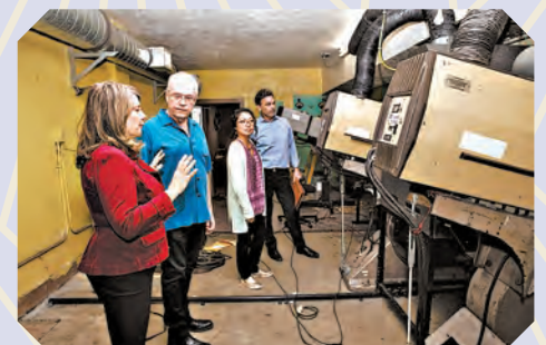
The project room high atop the Warner Grand's mezzanine contains equipment both modern (the large orange boxes in the back are digital projectors) and obsolete (the reels in the front right are film projectors and a film platter). All of the projection equipment is vintage and has been donated (the Super Trouper follow spots, from which the Abba song is named, are from the Dorothy Chandler Pavilion, and the film projectors are from the United Artists Four-Star Cinema on Wilshire, which has been closed). The equipment is in demand from collectors. A follow spotlight is in the very back.
