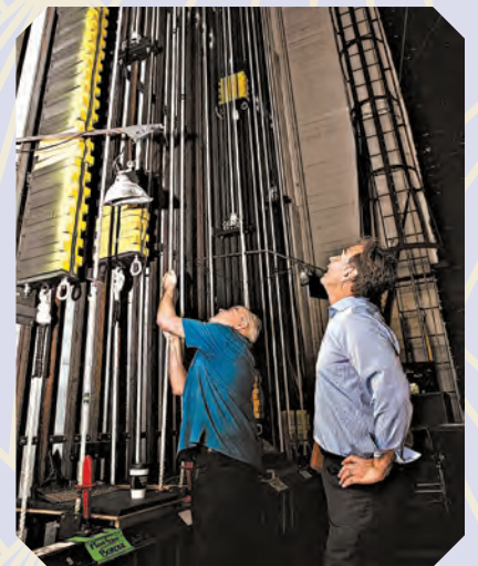
Lee Sweet, Theater Manager, shows Club CEO John Hawkins how the modernized rope pulley system works for scene changes.
