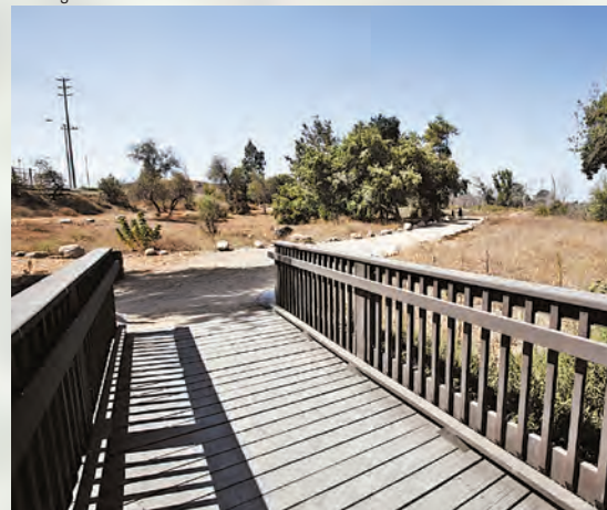
A bridge crosses over a small creek to the trail.
