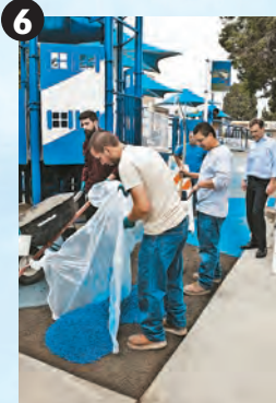
The new surface is poured in place.
