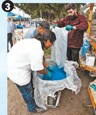
The crew prepares the new pour-in-place surface — a state-of-the-art combination of recycled rubber, coloring and glue. This kind of surface produces no abrasions to the skin of those who play on it.
