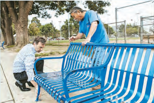
Benches: Dale checks to make sure the benches are stable, with paint and welds in good order. This one checks out.
