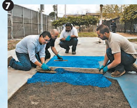
Smoothing and leveling the new surface with trowels before it hardens is critical.
