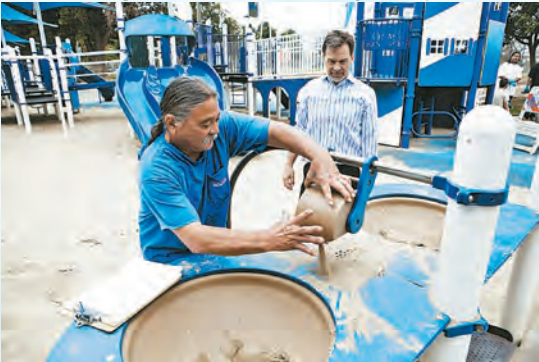
Sand scooper/sifter: This unit is in good shape.
