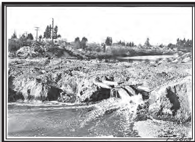
A broken sewer on Jefferson Street in West LA, before repairs, in November 1936.
