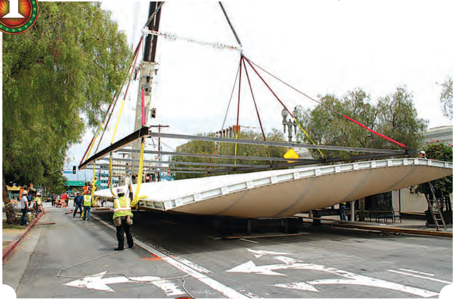
The mural shelter was delivered by truck onto Main Street...
