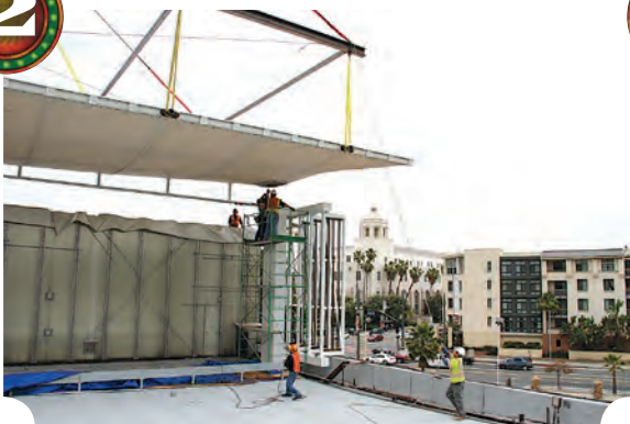
... lowered onto its massive supports on each side of the mural...
