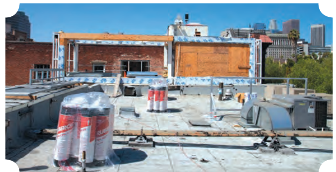
The viewing platform under construction.
