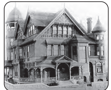
Circa 1890: The exterior of the mansion owned by businessman Leonard John Rose, on the southeast corner of Grand Avenue and Fourth Street. The lavish home, completed in 1888, was designed by Curlett & Eisen and cost approximately $50,000 to build.
