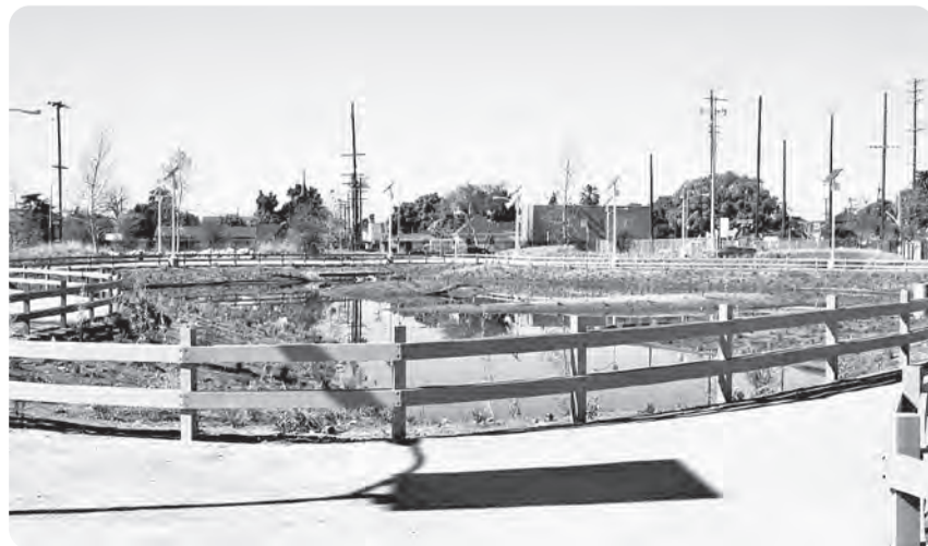
The water basin, walking path and surrounding vegetation.
