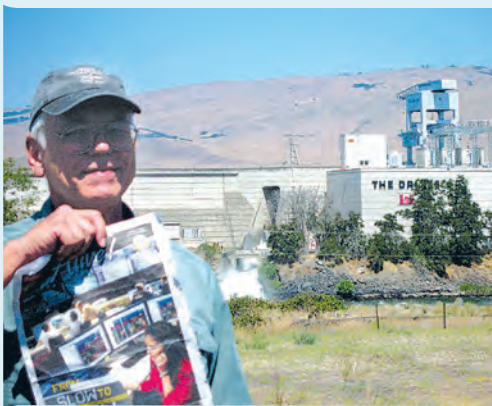
"This is The Dalles, a hydro generator on the Columbia River that supplies power to the Pacific DC Intertie transmission system that connects to Los Angeles, 846 miles away, the longest DC line in the USA."
