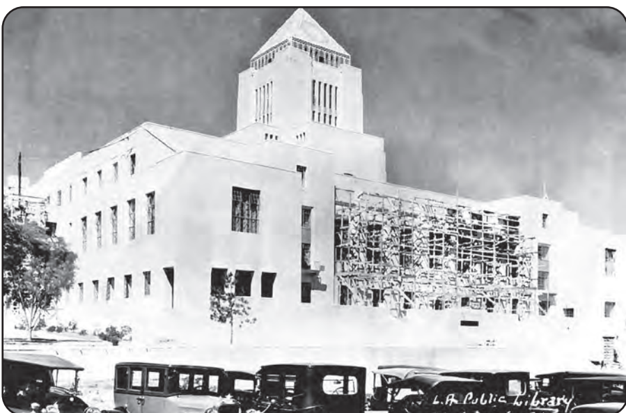
This 1926 photograph shows construction of the Los Angeles Public Library, located at 630 W. Fifth St. The view is looking at the southwest corner. The structure, which is almost complete, shows scaffolding along a portion of the south side. Several automobiles are parked at Savoy Auto Park, visible in the foreground.
