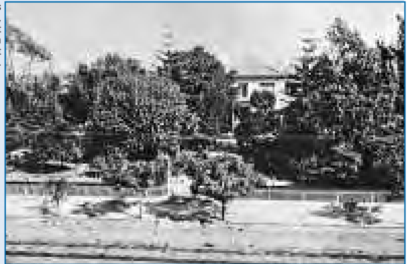
Cameron Thom's residence in 1886, at the southeast corner of Main and Third Street downtown.
